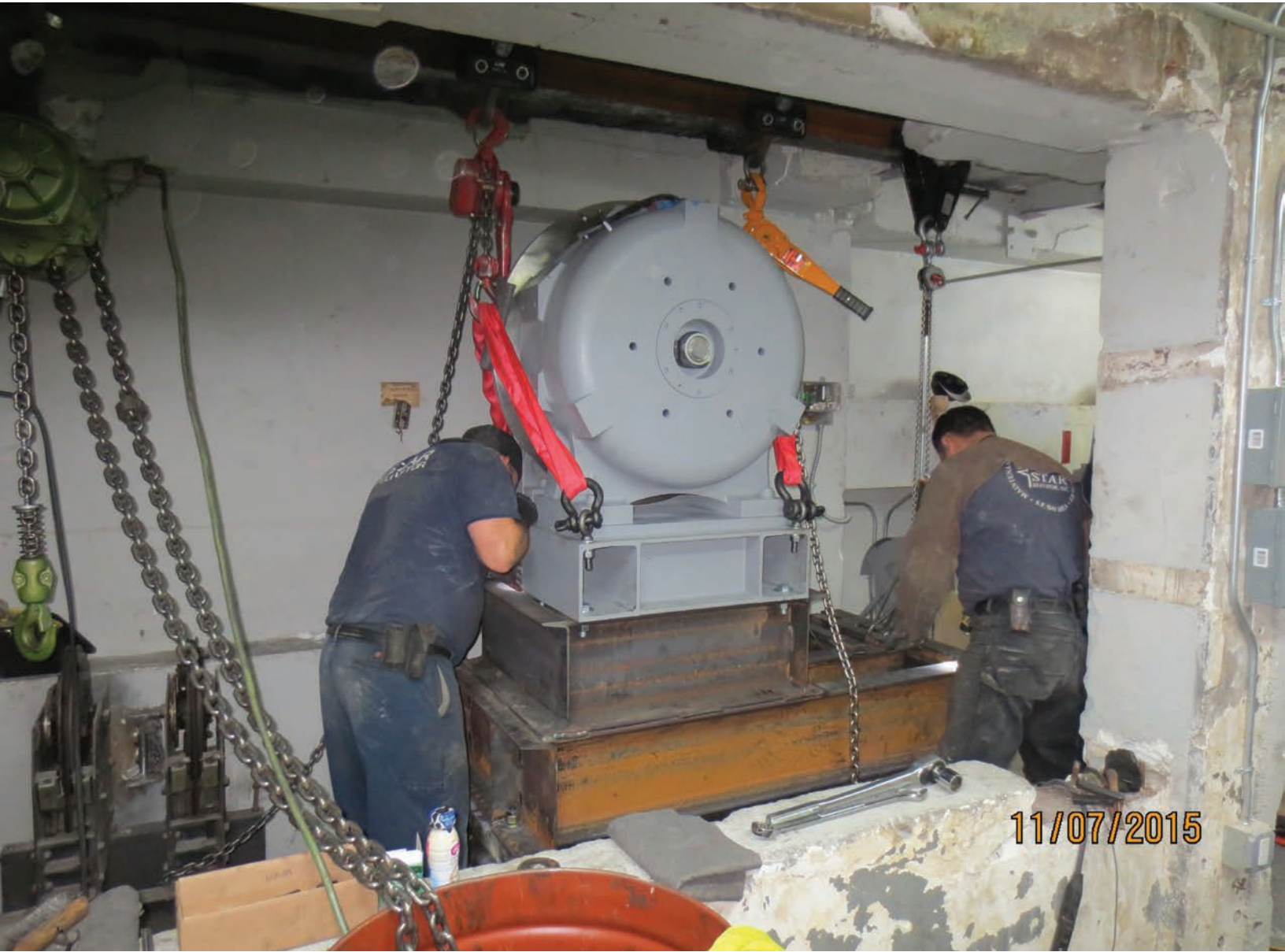
New equipment in overhead location.
